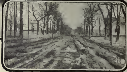
Typical Spring conditions on a soft-surfaced road
